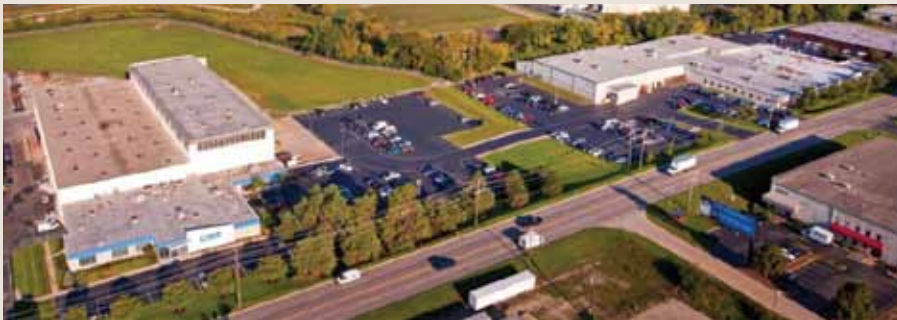
CSZ has two manufacturing facilities in Cincinnati, OH with world-wide sales and service.
